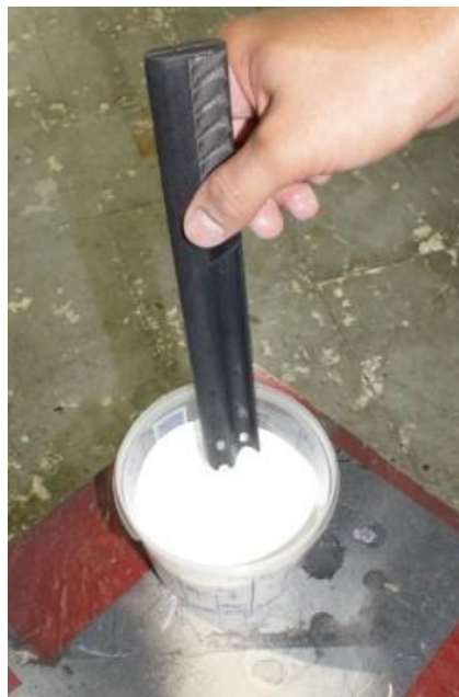
Figure 5.4 Mixing of painting colour
