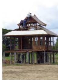
Phase 2 - Structuring and Roofing Phase
