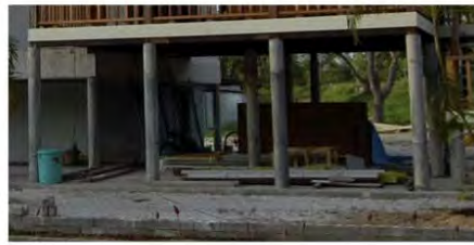
Phase 1 - Cement Foundation Phase
