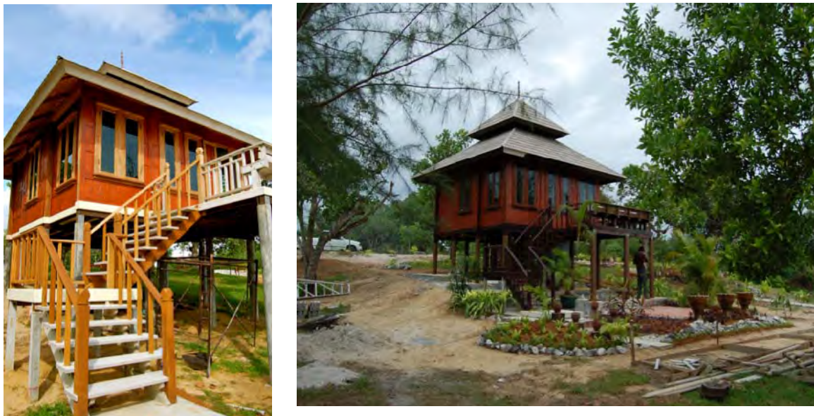
Figure 3-1. Example of Shera house.
