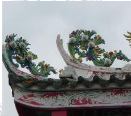
Figure 24 The swallowtails of main ridge and tails of ridges
