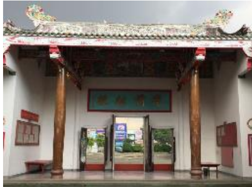
Figure 14 The inner of the head door of the ancestral hall of XCAT
