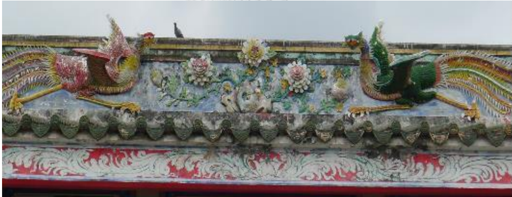
Figure 21 The Chaozhou trencadís of the double phoenix facing the peonies in the ridge of roof abdomen in the central segment
