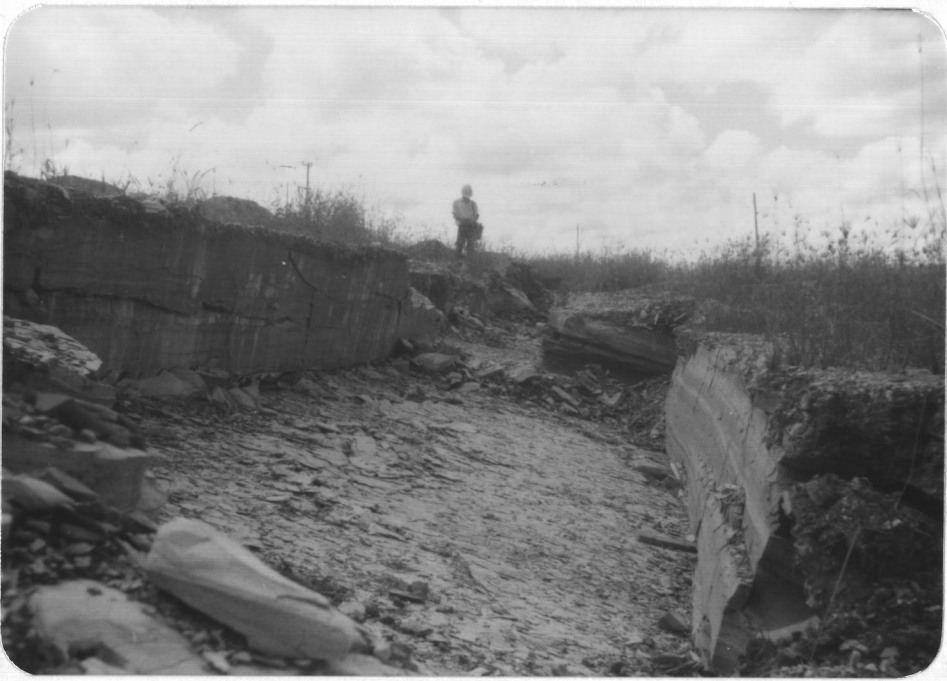
Figure 20. Separation of joint due to block slide in Subarea 5.
