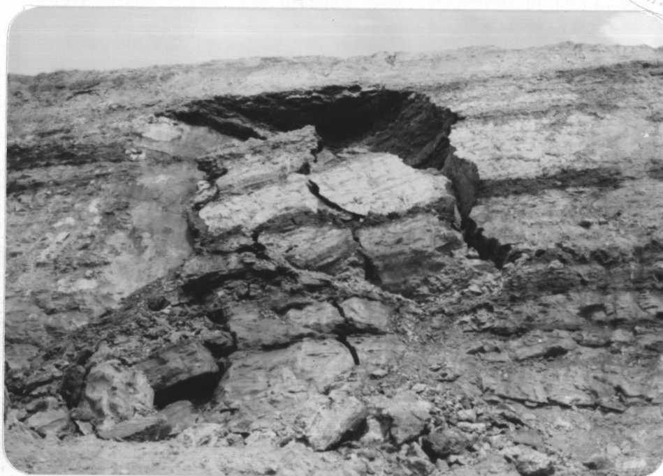
Figure 16. Local wedge failure of the northwestern flank slope in March, 1980.
