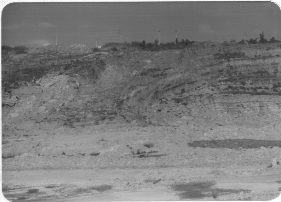
Figure 18. Landslide of Subarea 3 in August, 1981.
