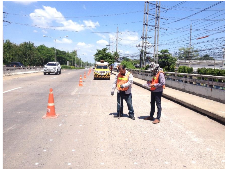
Figure 36 Sounding test on bridge deck
