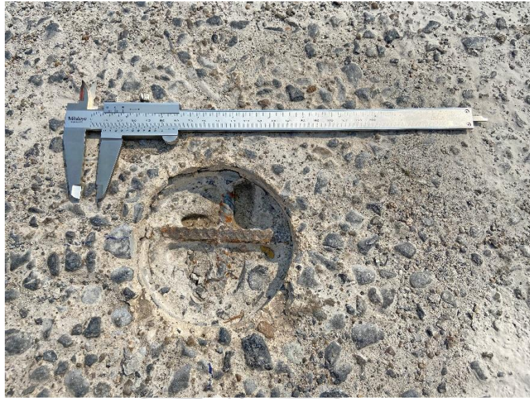
Figure 83 Steel surface on bridge span no. 3 at gridline K-L/1
