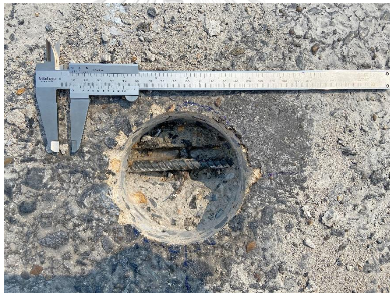
Figure 86 Steel surface on bridge span no. 7 at gridline L/5
