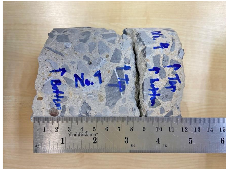
Figure 80 Concrete sample located on bridge span no.7 gridline E/2
