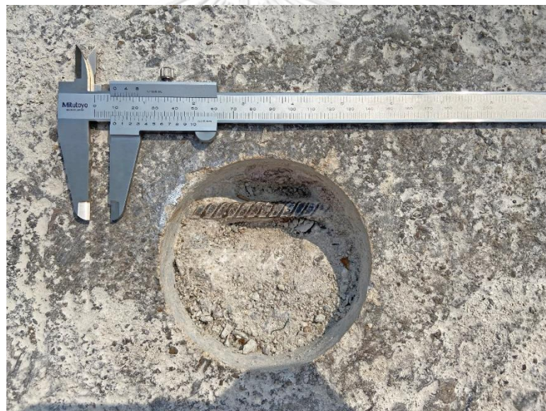
Figure 82 Steel surface on bridge span no. 1 at gridline I-J/3
