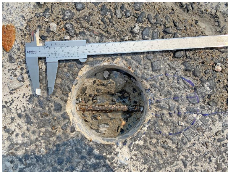
Figure 84 Steel surface on bridge span no. 8 at gridline H/3
