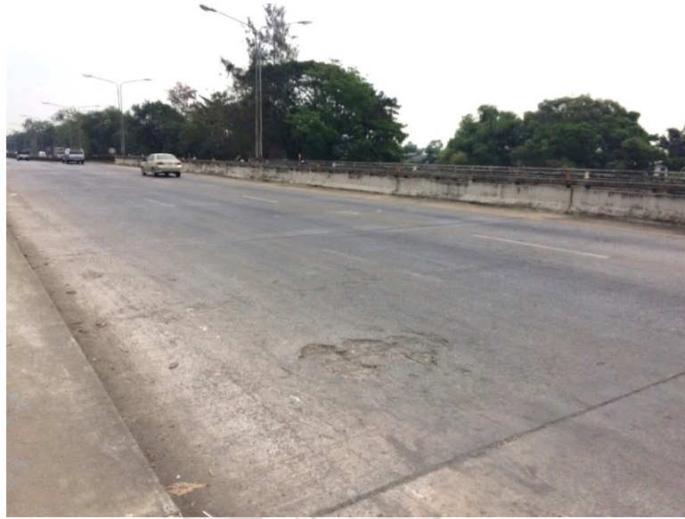
Figure 9 Klong 15 bridge on route 305 Rangsit-Nakhon Nayok (outbound side)
