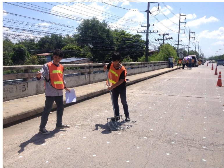
Figure 26 Chain drag test on bridge deck
