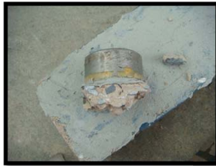
e) The appearance of damaged concrete after pull-off testing
