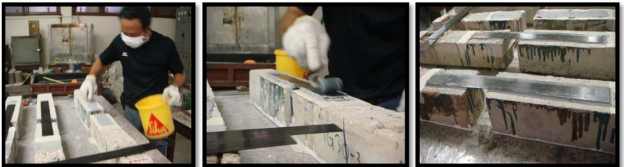
Figure 26 Attaching CFRP plate on concrete surface
