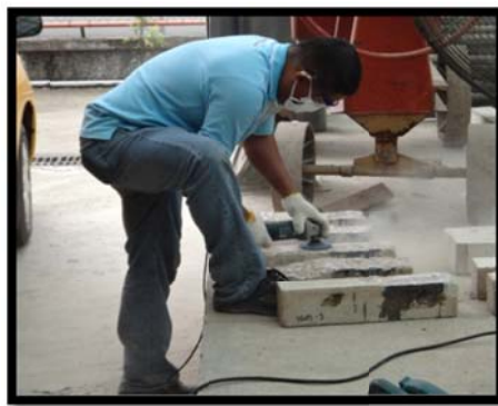
(a) Leveling concrete surface
