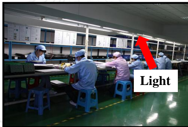
Figure 10 Lighting system in manufacturing
