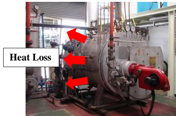
Figure 28 Heat losses from a boiler
