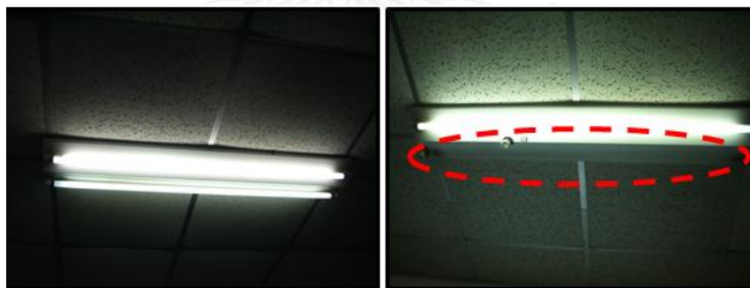
(a) Before removing light bulbs
