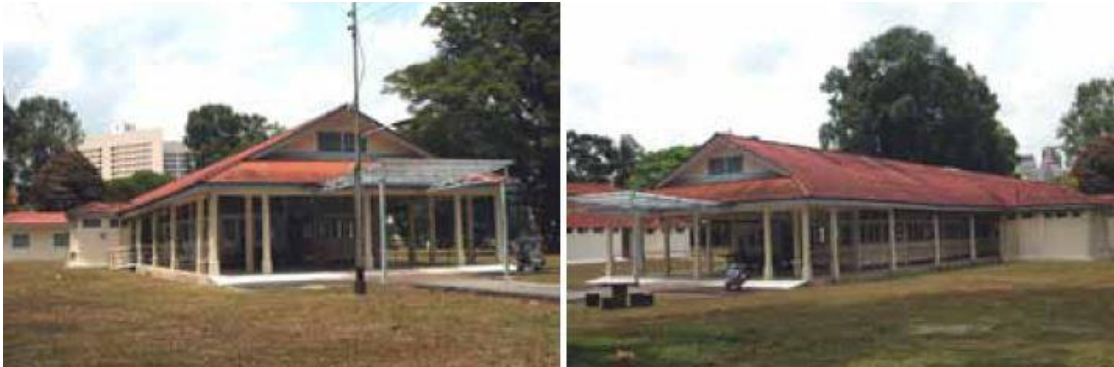
Figure 2.5 Single story Tuberculosis inpatient ward with windows on all sides allow for maximum natural ventilation
