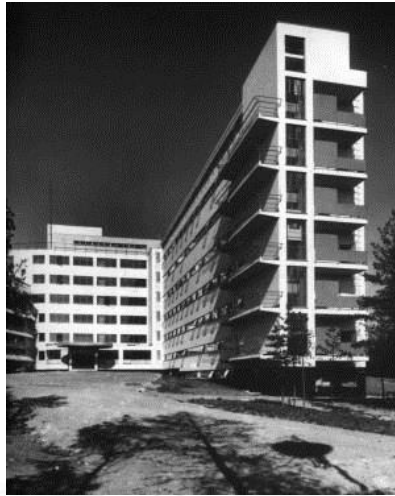
Figure 2.1 Exterior of the Paimo Sanatorium in Finland
