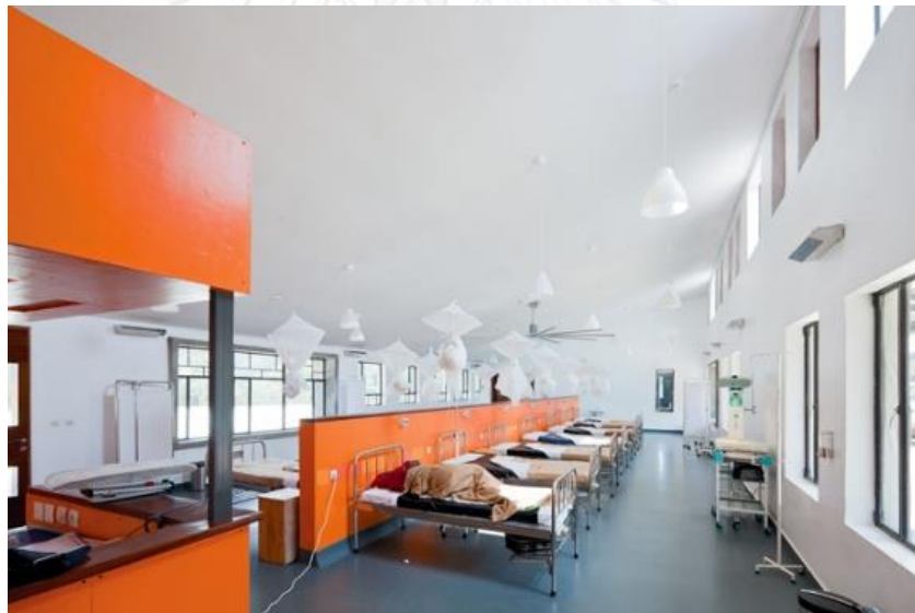
Figure 2.8 An interior of Butaro IPD ward. Tall ceiling with windows allows micro bacteria to rise up and diffuses through the top opening
