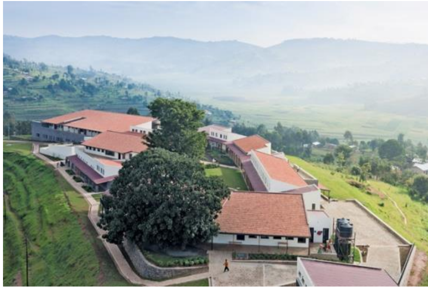
Figure 2.7 Aerial view of Butaro hospital exterior
