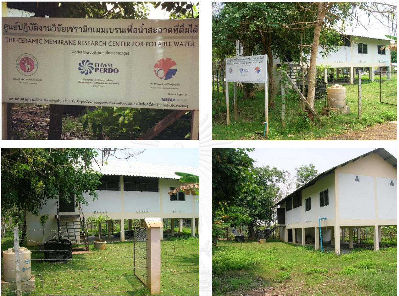
Figure B. 7 The Ceramic Membrane Research Center for Potable Water
