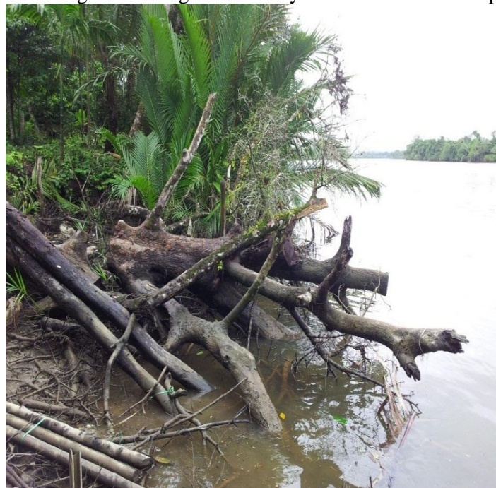
Figure 4: Mangroves destroyed and river back collapsed
