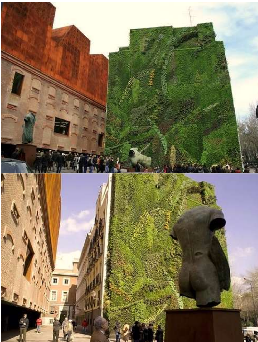
Green Vertical Garden (wall) in Madrid
