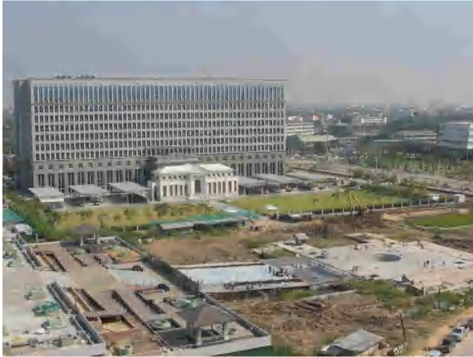
Figure 3.2 Picture of Office building of the Administrative Court construction
