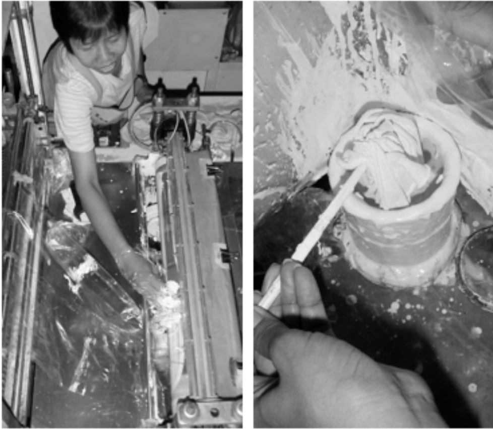
Figure 3.6.10: The processes of apply sealing liquid
