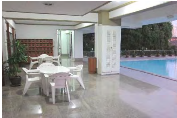
Image 5.8) Lounge area that requires upgrading.
