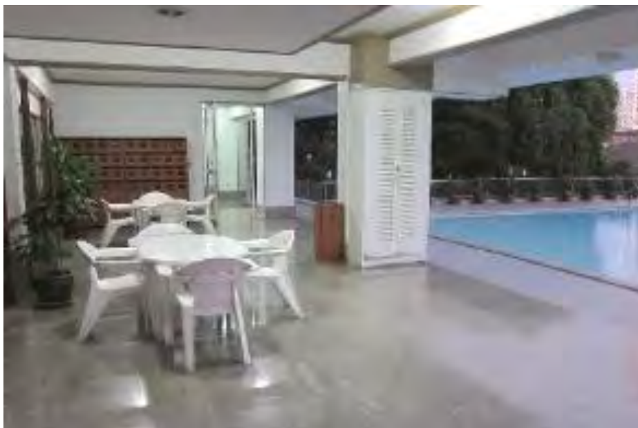
Image 4.7) Inadequate swimming pool furniture.
