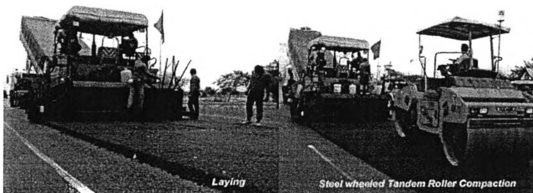
Figure 2.4 Laying and Steel wheeled Tandem roller compaction.
