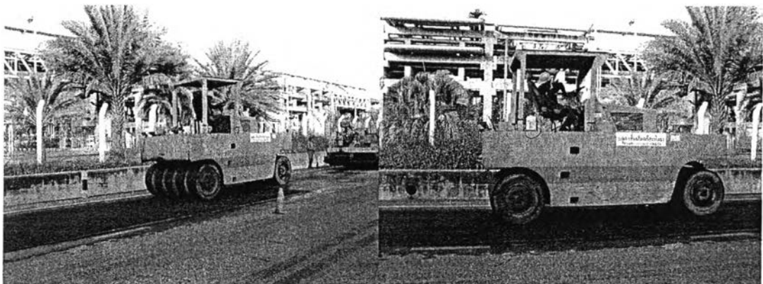
Figure 4.48 Static pneumatic tired roller (SAKAI TS200).
