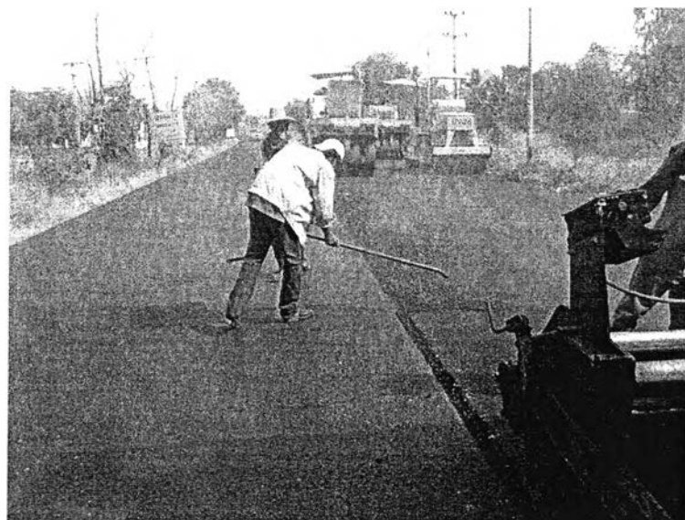
Figure 4.19 Equalize at edge joints.
