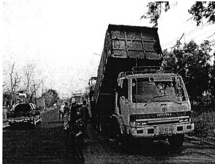
Figure 4.18 Asphalt concrete truck pour hot-mixed asphalt into paver.
