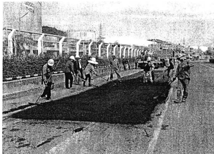
Figure 4.46 Equalize at edge joints.
