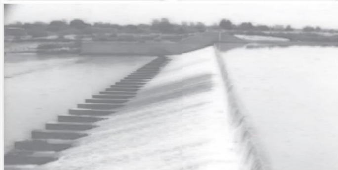
Thedaw Dam has emerged in Letpadan Township, Bago Division, thanks to collective endeavours of the people and the Tatmadaw.
