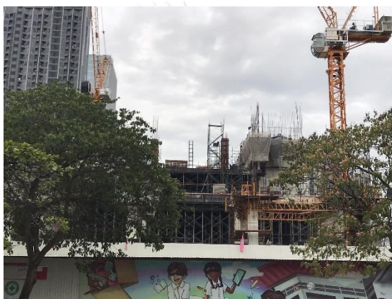
Figure 7.36 Chulalongkorn University Demonstration Secondary School construction project.
