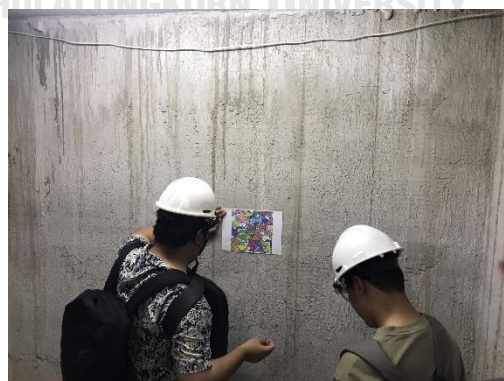
Figure 7.41 Installation of markers in the construction project.
