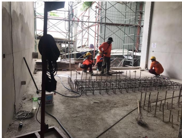
Figure 4.10 Example of the number of workers and construction activities on day 2.
