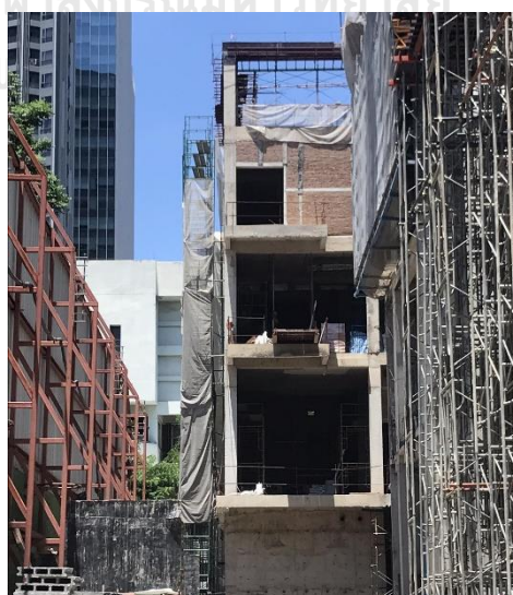
Figure 7.37 The construction project for an engine building.
