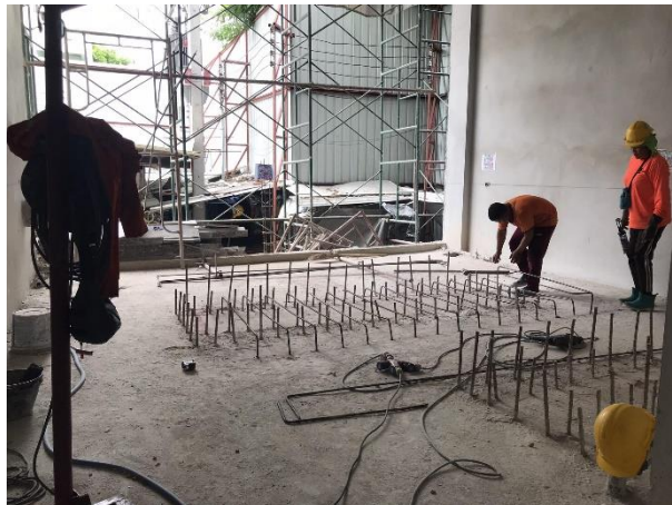
Figure 4.9 Example of the number of workers and construction activities on day 1.
