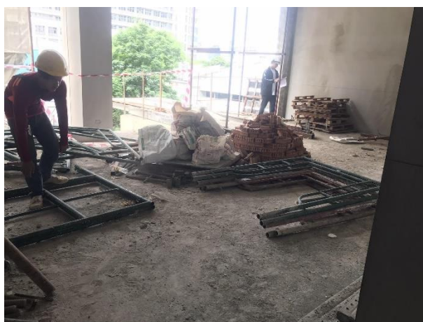
Figure 4.11 Example of construction worker in material handling activity.
