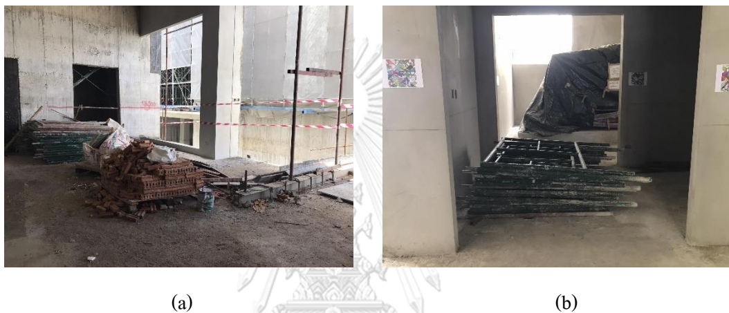
Figure 7.29 Example of the temporary material area in the construction project.
