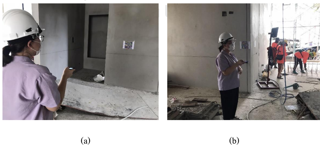
Figure 7.11 Measure the distance using the Matal Laser Distance meter in case study 2.
