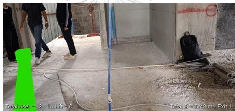
Figure 7.43 Example of the output of the proposed system for respondent number 1 in the case of the 1 st floor.
